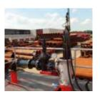
4 The pump (with seal) is hung in the hoisting cable and inserted through the T-piece into the pipe.
