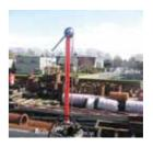
3 The winch is bolted onto the T-piece top flange.
