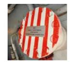
1 Removal of the blind flange gives access to the sounding or vent pipe.
