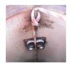
5 Once the required depth is reached the hoisting cable is firmly anchored using cleats and the winch is removed.
